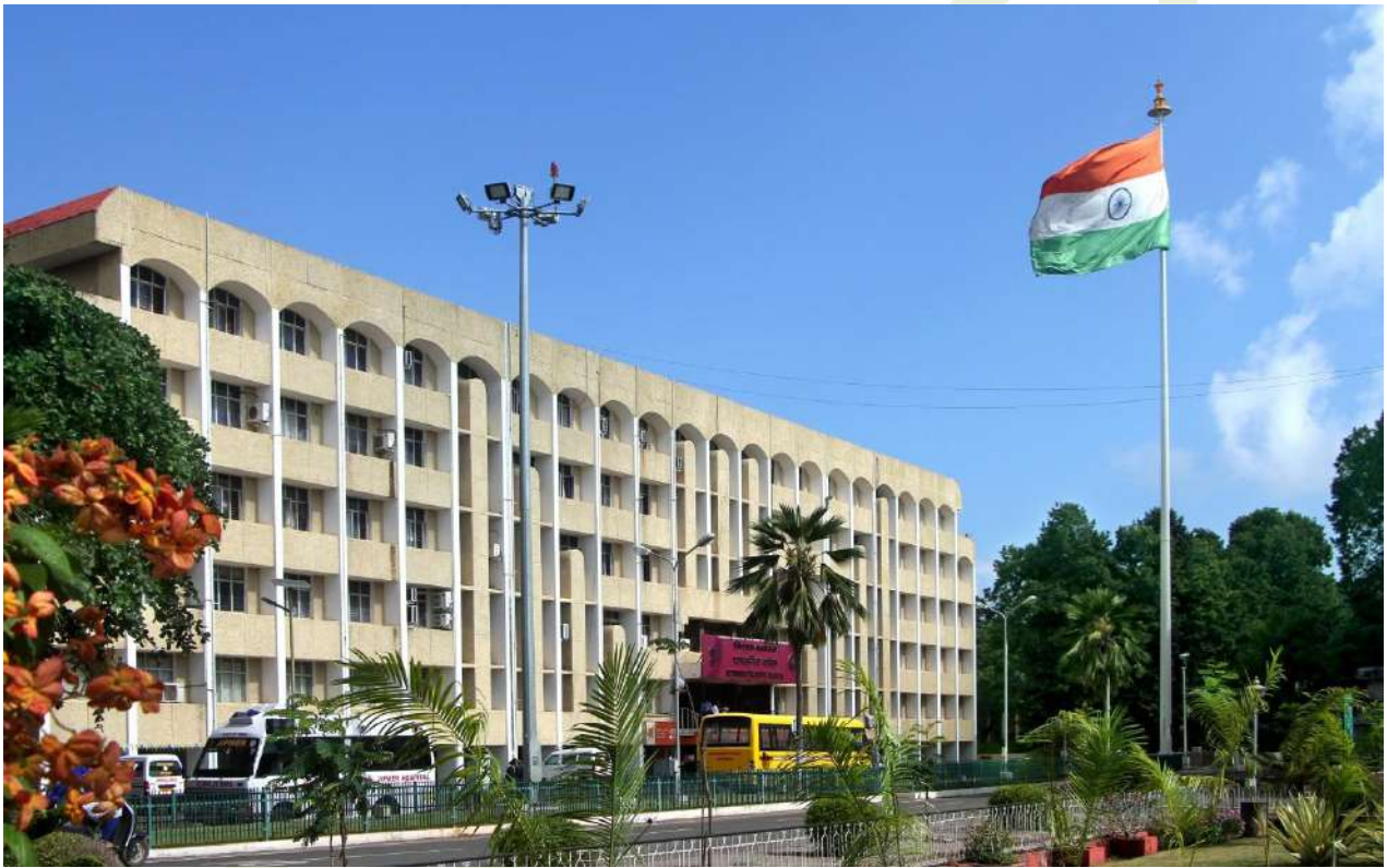
Administrative Block, JIPMER Puducherry
